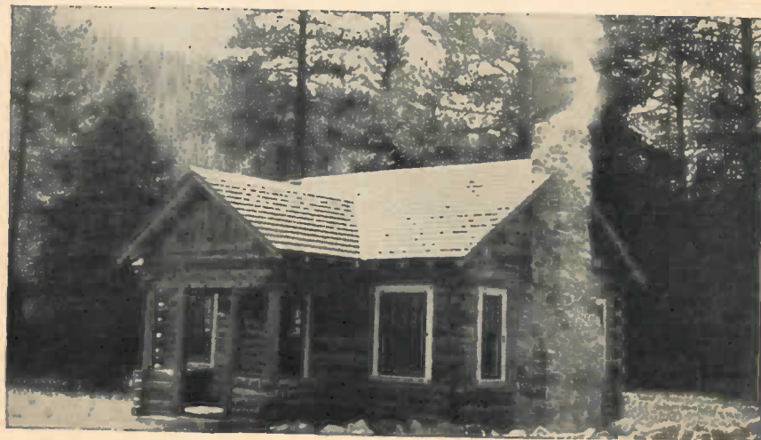
FIGURE 28.—Fine example of milled-log construction—ranger's dwelling, Whitman National Forest, Oreg.
