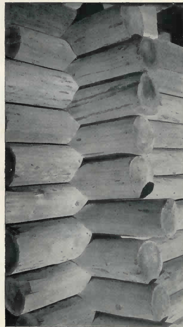
FIGURE 2.—The round-notch or saddle corner. This is an unusually fine example of scribing and fitting logs together. The square-cut logs have yet to be dressed and shaped with the ax to give them a pleasing appearance.
