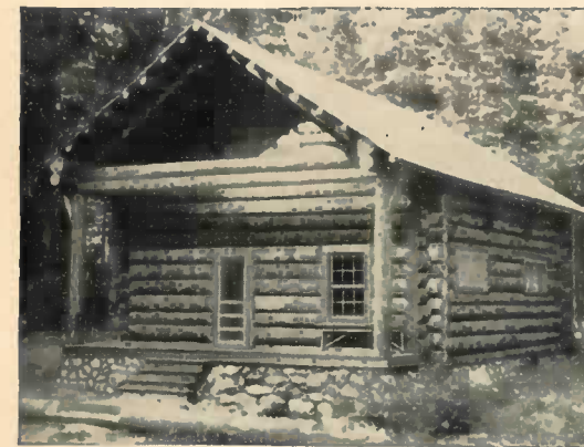
LOG BRACKETS UNDER EAVE SHAKES SUPPORT INCREASED OVERHANG
