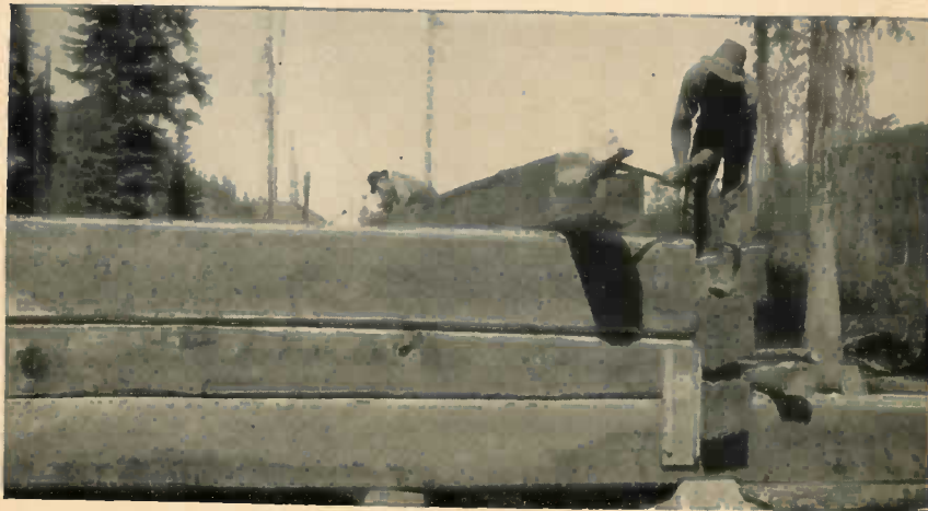
FIGURE 29.—Framing hewed timbers.
