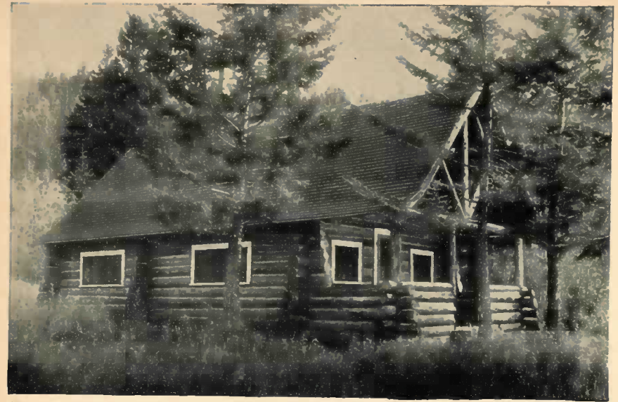
FIGURE 32.—A useful type of modern log dwelling—ranger station, Gallatin National Forest, Mont.
