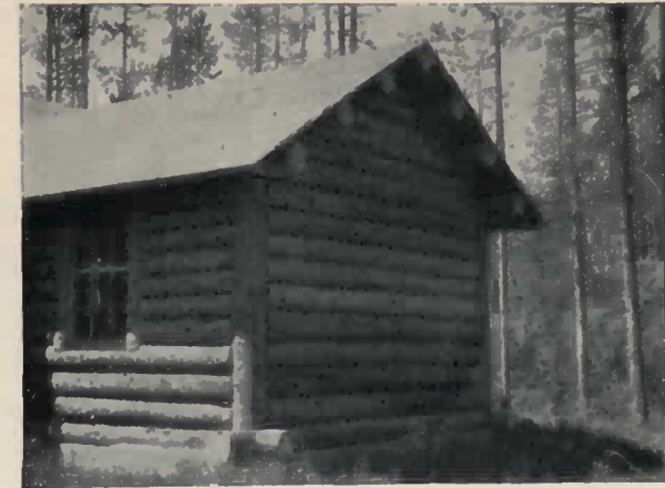
UPRIGHT OR GROOVE AND TENON CORNER
