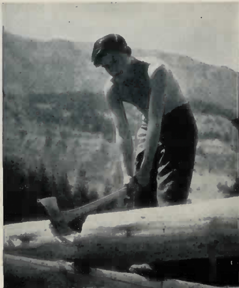
FIGURE 5.—Chopping the notch in a saddle corner.
