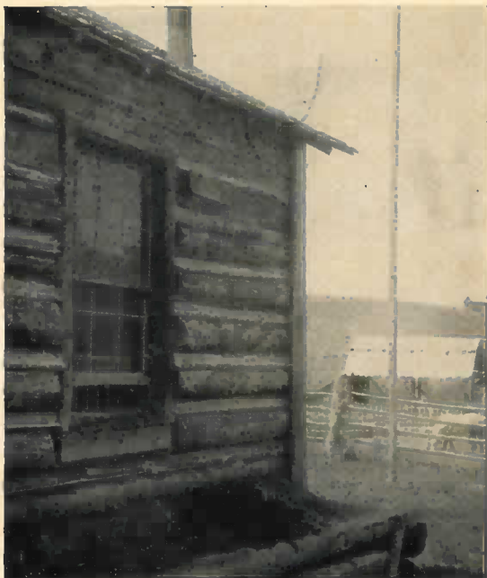
FIGURE 26.—Wood daubing strips.
