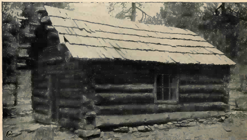
FIGURE 35.—Early types of log structures built by the U. S. Forest Service in the West. A, Ranger station, Gallatin National Forest, Mont.; B, ranger's dwelling, Nezperce National Forest, Idaho; C, log cabin in Arizona.
