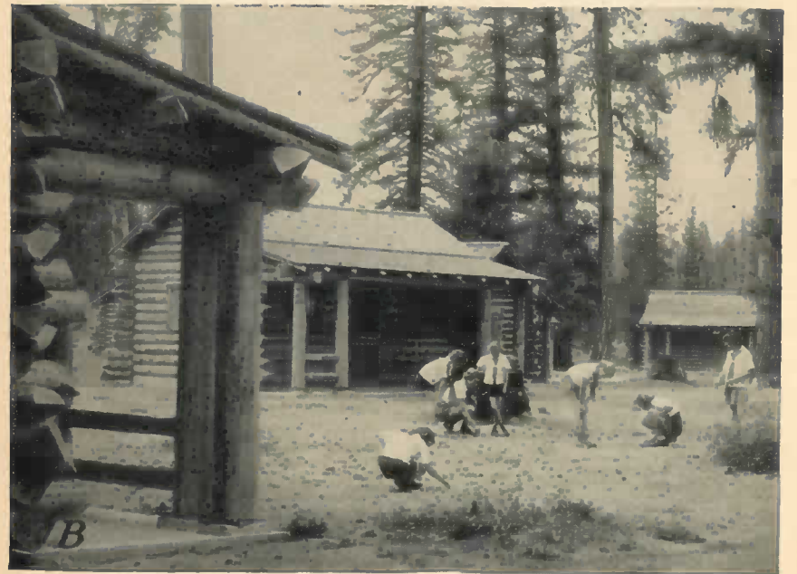
FIGURE 34.—Organization camp at Seely Lake showing log work in greater detail. A , Entrance wing; B , cabin group. Note the wedges under porch post to provide for settling of walls. Wedges are gradually driven out as necessary.
