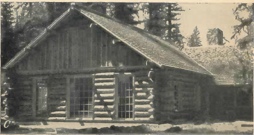
FIGURE 33.—Modern structures showing effective use of log construction in recreation buildings on national forests in Montana. A , Dude ranch; B and C , recreation and mess hall, Seely Lake.
