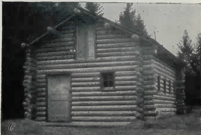
FIGURE 3.—Ranger station, Gallatin National Forest, Mont., illustrating effective use of round-notch corners. A, and B, Dwelling under construction; C, barn.
