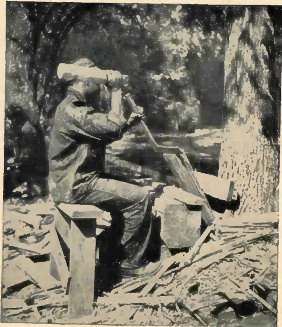
FIGURE 20.—Splitting shakes with the froe.
