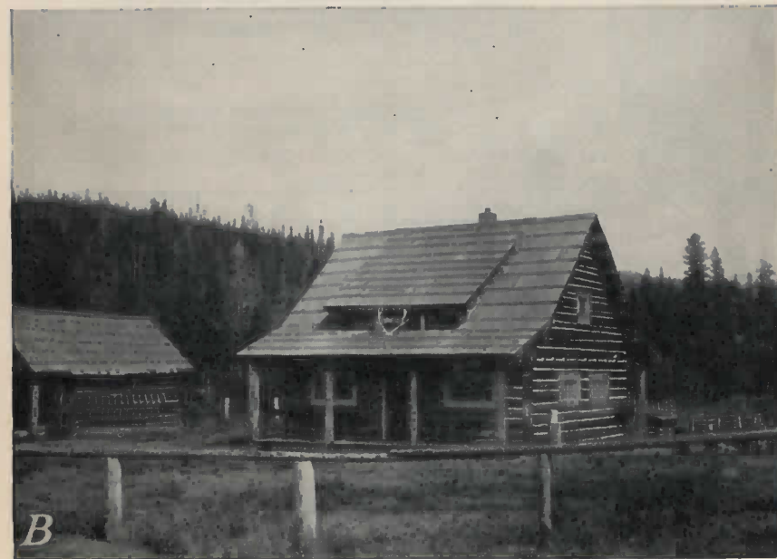
FIGURE 7.—Ranger Station, Lolo National Forest, Mont. Note the meticulous construction of box corners.
