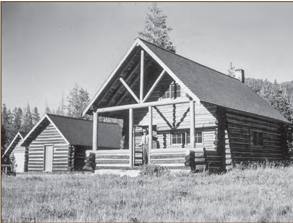
Figure 204—A simple king post truss constructed of logs supports the porch of the cabin at the Stolle Meadow Guard Station (Boise National Forest, Intermountain Region). The cabin has a cedar shingle roof. This photo was taken in 1939, not long after the builders constructed the cabin. The cabin still is in use today.
