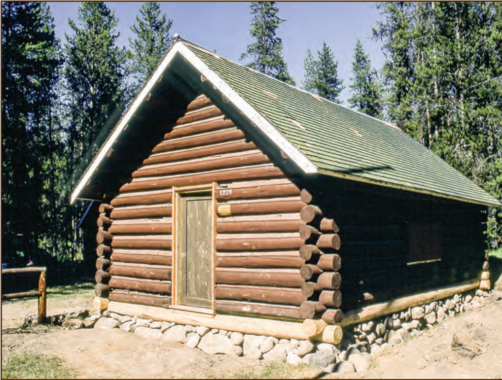
Figure 10—The people who restored this pre-1914 storage cabin at the Stolle Meadows Guard Station (Boise National Forest, Intermountain Region) carefully replaced the dry-laid stones between the rock corner piers after they replaced the sill and spandrel logs.
