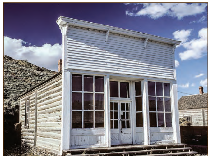
Figure E41—The owner added a false front consisting mainly of windows and clapboard siding to this log building in South Pass City, WY, to make it look more substantial and prosperous. Photo © Andrew Gulliford; used with permission.
