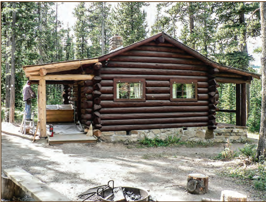
Figure 325—The King's Hill Cabin (Lewis and Clark National Forest, Northern Region) had an ongoing ice problem at the back stoop because of refreezing melt water running off the uninsulated roof. The cabin now has a new back porch to shield the back stoop from ice and to also provide an accessible entrance to the building. The addition of the stylistically compatible porch ensures the cabin's continued use in the winter. The porch is clearly differentiated from the original construction by the wooden walkway and the concrete (rather than stone) column supports.
