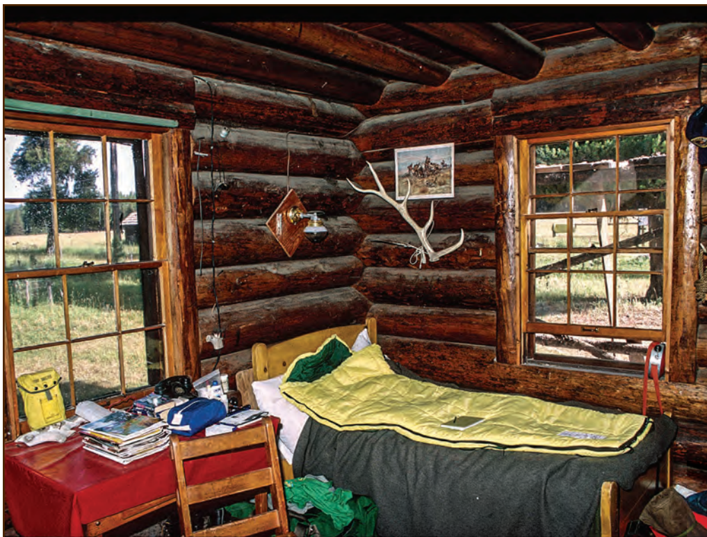
Figure 47—The single-hung windows in this cabin are newer than the rest of the cabin. Telltale evidence includes the window manufacturing style and the double log trim above the windows. Someone probably used the double trim to mask the gap between the shorter new windows and the logs that were cut for the taller original windows. These changes are typical of evidence that you may find in a structure that is relatively well cared for.
