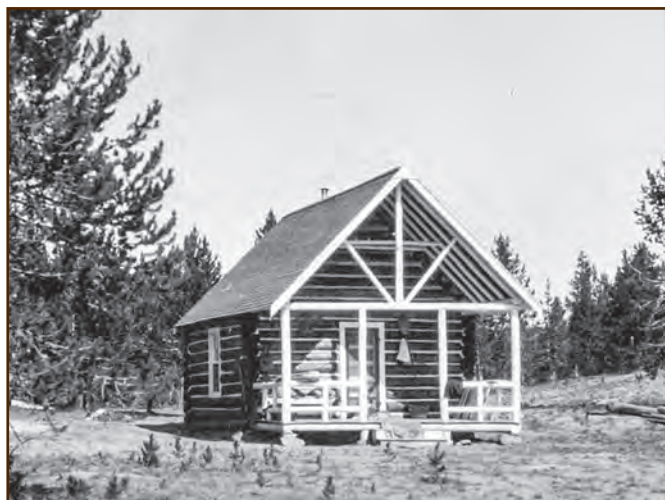
Figure E10—The builders constructed the assistant ranger's house at the Landmark Ranger Station on rock piers in 1936. The Landmark Ranger Station now is a seasonal-use guard station on the Cascade Ranger District in central Idaho (Boise National Forest, Intermountain Region).
