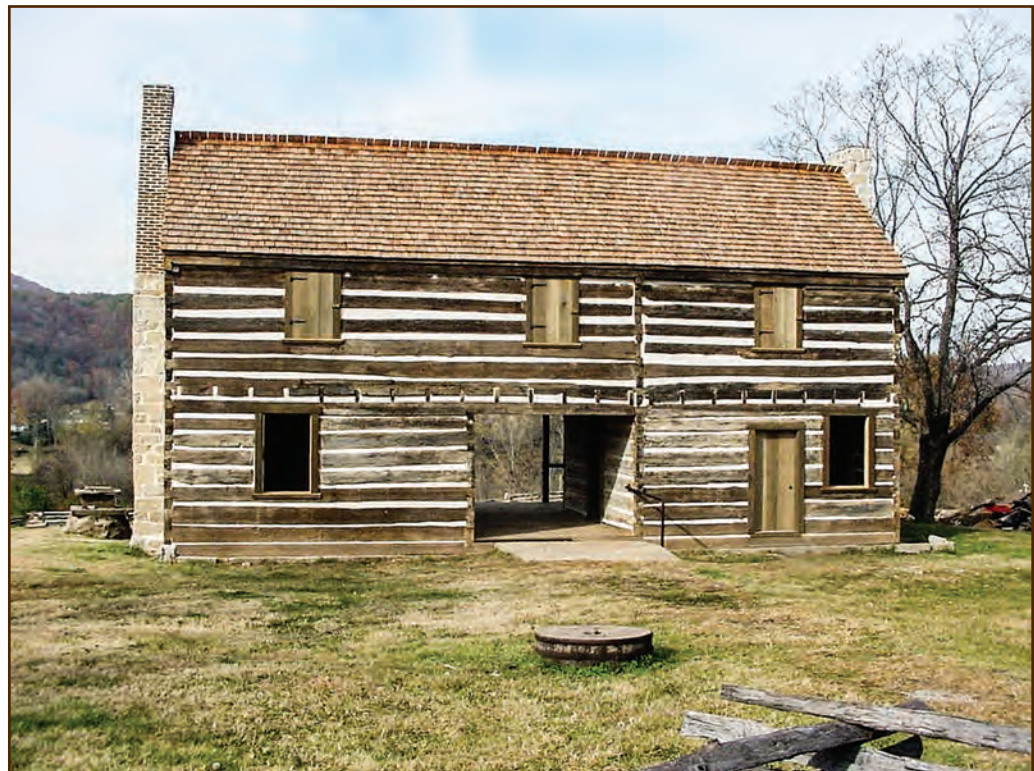
Figure 308—The Wolf House in Norfolk, AR, built in 1829, has masonry fireplaces and chimneys on each end. The builders constructed the original chimneys of local stone. Someone apparently reconstructed the top of the chimney on the left side of the building with brick at some point after 1960; a photo from 1960 shows the chimney completely constructed of stone.
