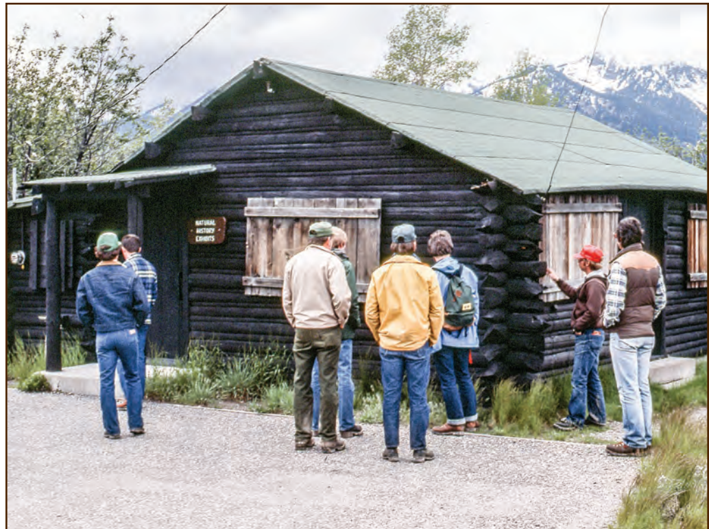
Figure 215—This early 20th-century log cabin in Grand Teton National Park has asphalt rolled roofing, just as it did originally. It now houses natural history exhibits.
