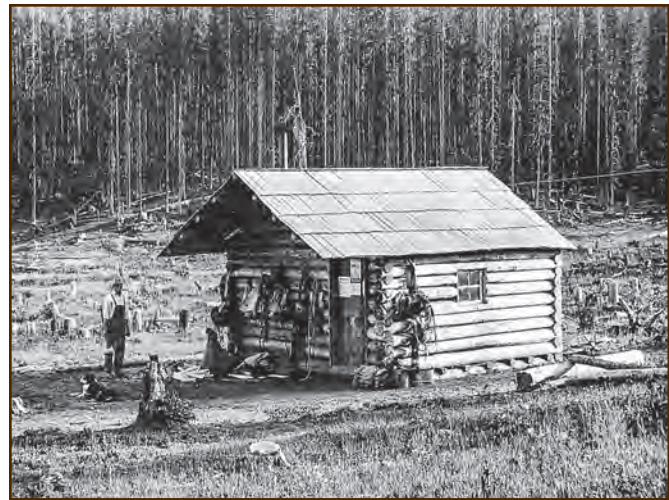
Figure E9—The log sleepers that support the Clearwater Springs Ranger Station cabin are clearly visible under the log floor joists in this photo. The builders constructed the cabin in 1913 and used it as a summer station in the Blue Mountains (Pomeroy Ranger District, Umatilla National Forest, Pacific Northwest Region).
