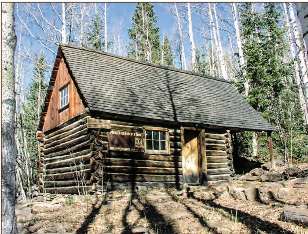
Figure 6—The Jubilee Guard Station is a one-and-a-half-story log cabin built in 1905 in the Escalante District of the Dixie National Forest, Intermountain Region. Located at an elevation of 9,800 feet on the Aquarius Plateau in southern Utah, it's one of the oldest remaining guard stations in the State.
