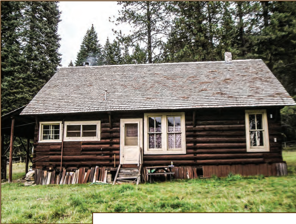
Figure 213—Roofers used shakes that matched the original roofing to reroof the Office/ Cookhouse building (Moose Creek Wilderness Station, Nez Perce National Forest, Northern Region). This photo shows the north side of the building.
