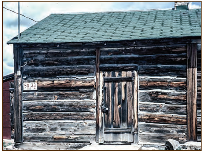
Figure E21—The stage stop in Virginia Dale, CO, has a post and beam structure with stacked log infill walls. The original roof was cedar shingles.
