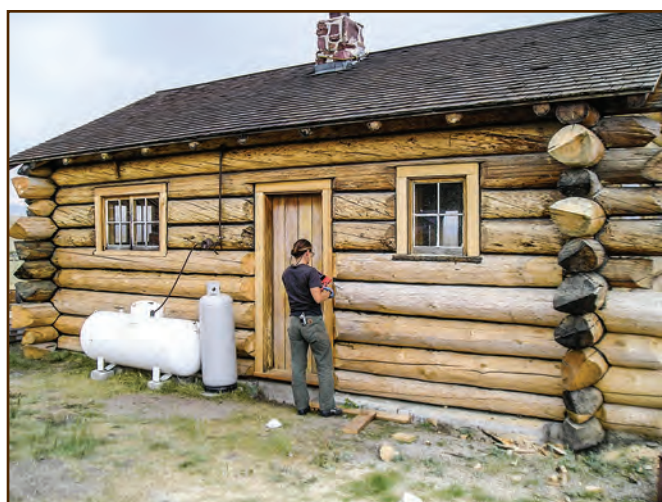
Figure E37—The tar daubing on the 1935 Horse Prairie Guard Station (Beaverhead-Deerlodge National Forest, Northern Region), a fairly common daubing material choice in the Northern Region during that time period, has the effect of accenting the joints between logs.
