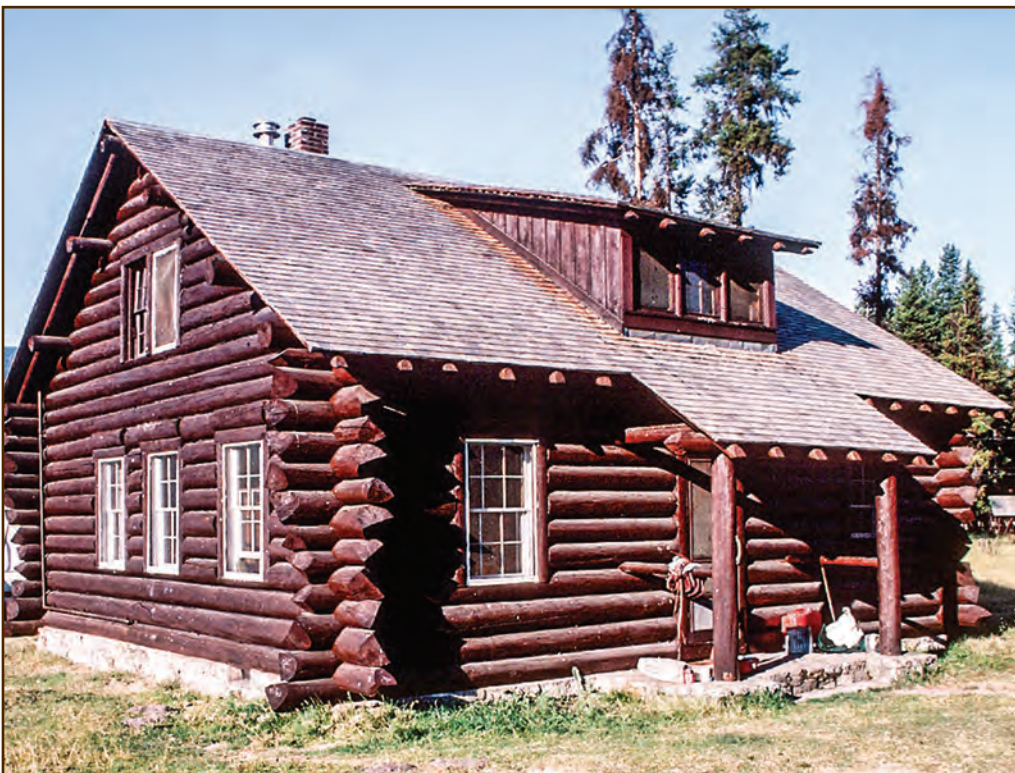
Figure 256—The shed roof dormer on the back of the Big Prairie Ranger Station (Flathead National Forest, Northern Region) has flashing at the base, sides, and top. The roofers installed base flashing where the lower side of the dormer meets the roof. The board and batten siding on the sides of the dormer covers most of the step flashing. The roofers also installed flashing at the transition between the top of the dormer roof and the main roof (not visible in the photo).
