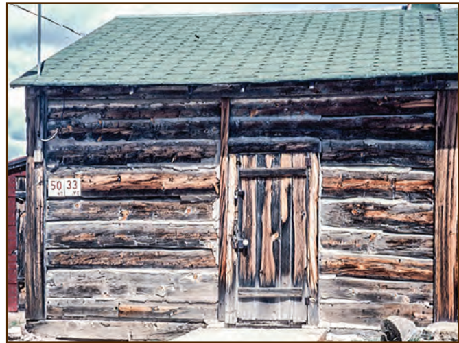
Figure 229—This cabin has an interlocking asphalt shingle roof. Builders have used this interlocking pattern since the late 1920s and still commonly install it on new buildings, particularly in high wind rural areas, because of its wind resistance. An interesting detail on this roof is the bent-over shingles at the roof eaves that function as a sort of inexpensive, integral drip edge.
