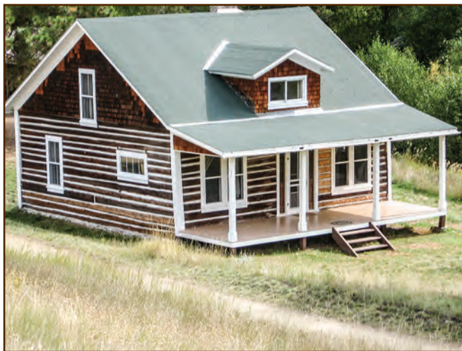
Figure 228—Builders constructed Hogback Cabin (Lolo National Forest, Northern Region) between 1913 and 1915 using rolled asphalt roofing. They used metal flashing all around the dormer and at the transition between the main roof and front porch roof.
