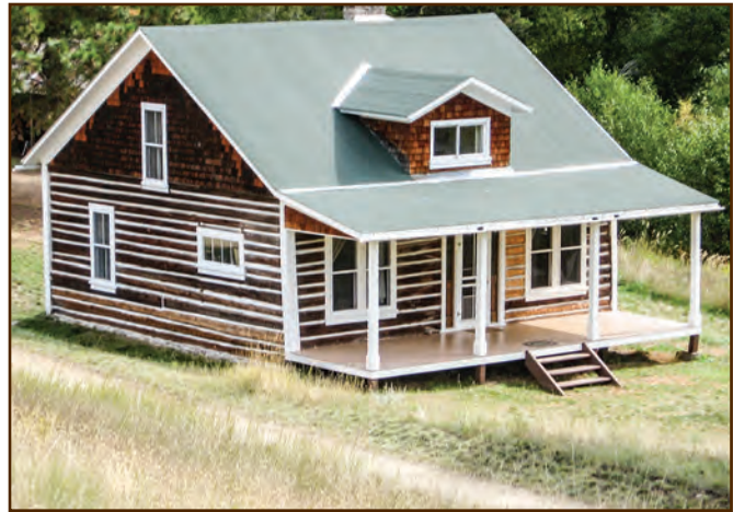
Figure E49—The Hogback cabin (Lolo National Forest, Northern Region) has unusual vertically applied asphalt rolled roofing. This photo shows new roofing that is identical to the original roofing.
