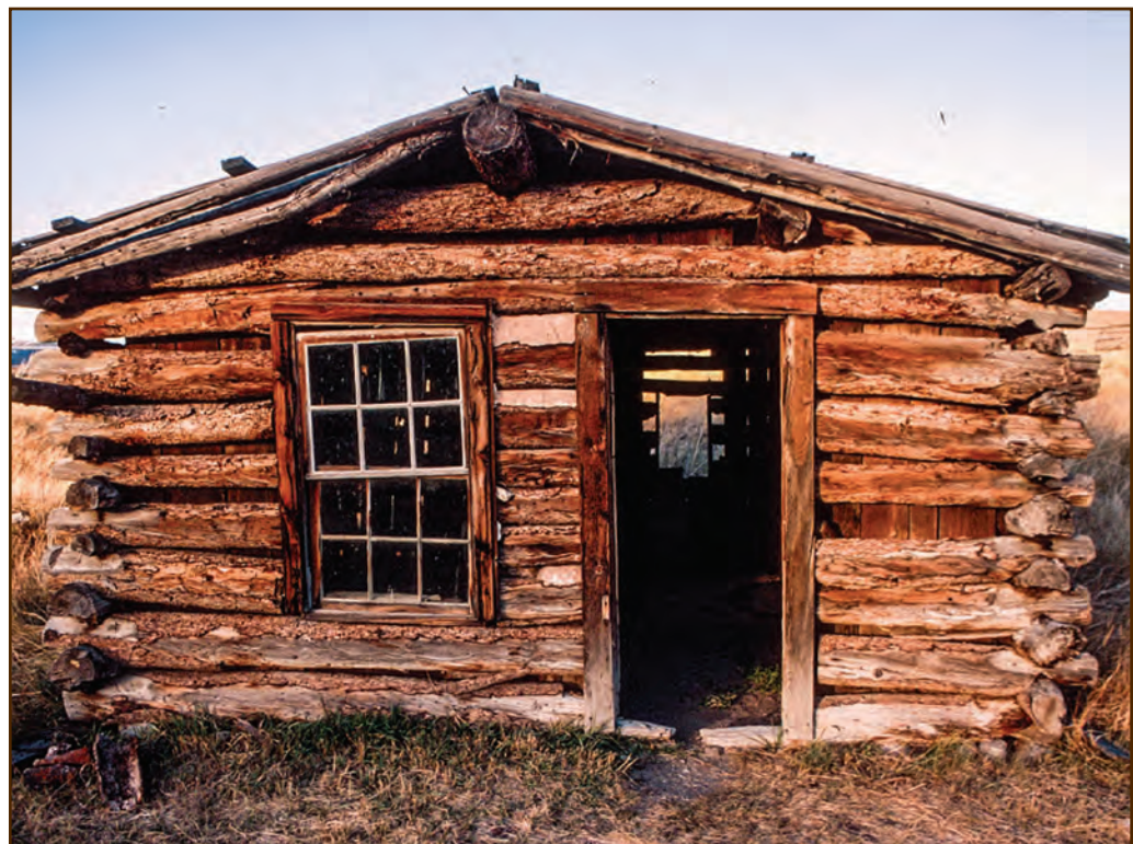
Figure 77—The builders constructed this small cabin on log sleepers laid directly on the ground. Despite the relatively dry climate, the sleepers have almost entirely rotted away, and the sill and spandrel logs have now begun to melt into the dirt also.
