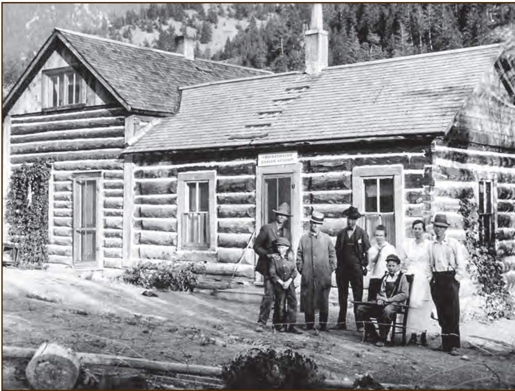
Figure 15—The builders enlarged Checkerboard Ranger Station (now within the Helena Ranger District) of the Helena National Forest, Northern Region, by adding a two-story log wing with a roof running perpendicular to the original log building.
