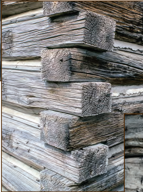
Figure E15—A square-notched cabin corner.
