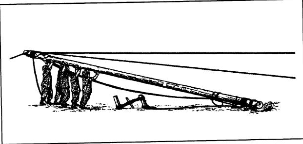
Figure 5-2. Erecting a gin pole
