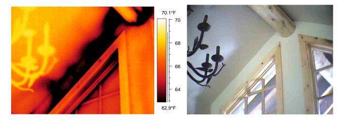
Figure 19 & 20. - Infrared cameras reveal substantial cooling during depressurization both around the ridge beam log and also at the sloped interface between the drywall and vaulted ceiling. Note that large openings existed between the log wall and roof soffit immediately opposite this image. These openings were permitting substantial air infiltration.
