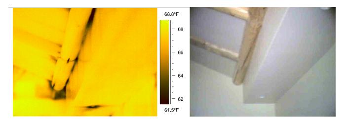
Figure 23 & 24. – Air infiltration observed as cooling at the end of log beam where it penetrates through the exterior wall, along the length of the beam at the interface with the drywall and at actual splits in the log itself.
