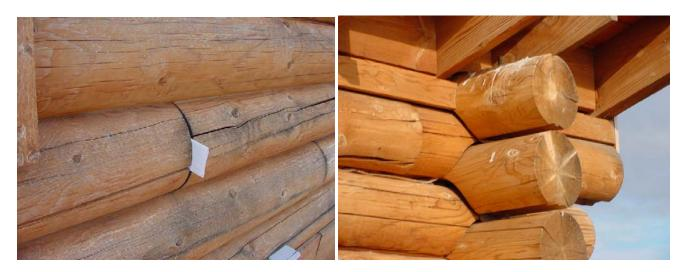
*Figure 3.* Open / un-sealed butt joint between logs. *Figure 4.* Open / un-sealed corner and successive joinery between logs.
