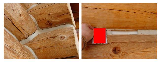
Figure 5. - Adhesively failed chinking at wood-to-wood log joinery. Figure 6. – Failed and missing chinking with insulation between logs at horizontal wood-to-wood joinery.
