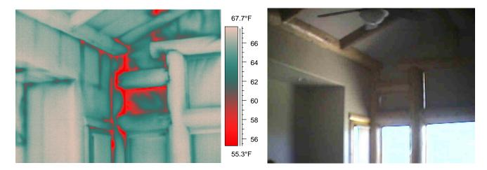
Figure 9 & 10. - Extensive air infiltration at wood-to-wood joinery in log assembly.
