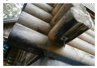
Figure 13: Typical connection with threaded rods through the logs
