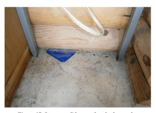
Figure 17: Ice-cream lid trapped under bottom log
