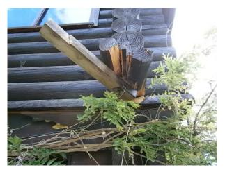
Figure 31: Crushing of bottom log
