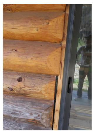
Figure 18: Localized sliding of logs
