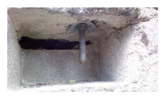
Figure 28: Bent washer in concrete pocket
