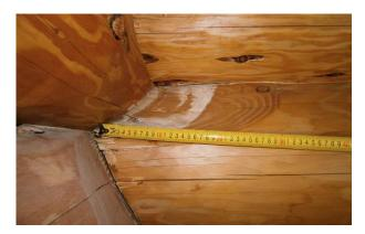
Figure 42: Permanent deformation in corner area
