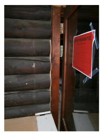
Figure 19: Localized sliding of logs
