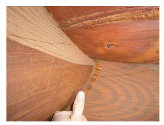
Figure 22: Sliding of the logs at corners
