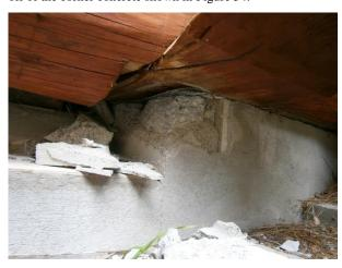
Figure 34: Cracking and spalling of concrete due to large compression forces
