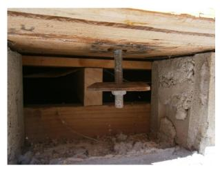
Figure 27: Fractured tie rod
