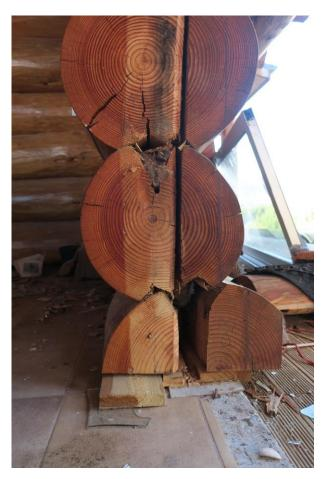
Figure 47: Splitting of bottom log
