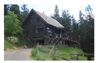
Figure 4: Two storey log house on slope with pole foundation
