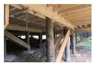
Figure 8: Pole supports with diagonal sub-floor bracing
