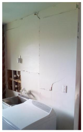
Figure 36: Typical cracking of gypsum plasterboard
