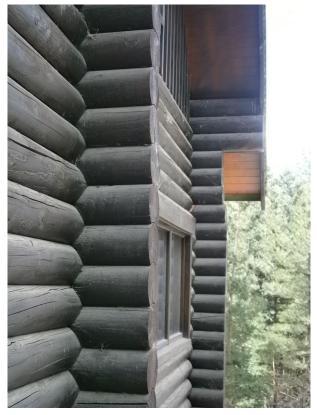
Figure 20: Sliding of logs resulting in residual drifts of the house
