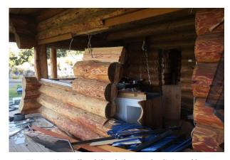
Figure 50: Wall stability failure and splitting of logs
