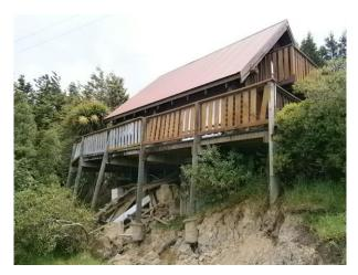
Figure 11: Two storey log house on slope with pole foundation with slope stability failure
