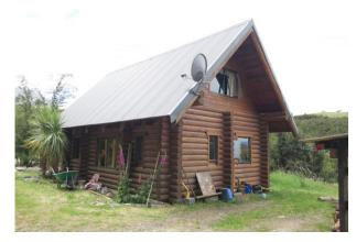
Figure 3: Two storey log house with slab on grade foundation
