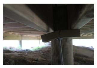
Figure 32: Failure of timber anchorage block
