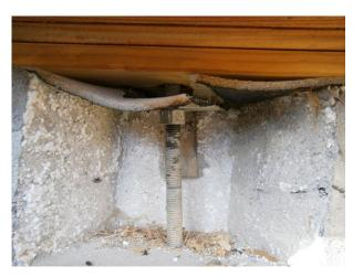
Figure 45: Yielding failure or fracture of tension rod
