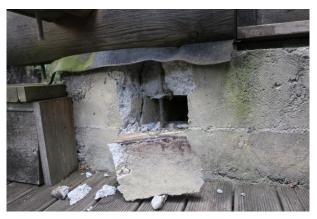
Figure 26: Damage to pocket in concrete foundation due to missing reinforcement
