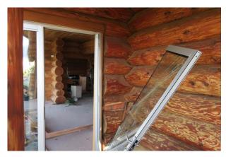
Figure 53: Typical damage to doors and windows due to large horizontal deformation
