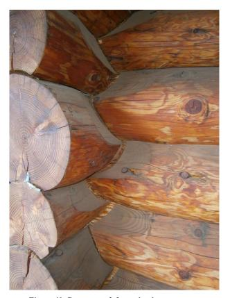
Figure 41: Permanent deformation in corner area
