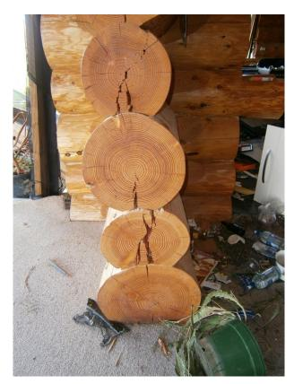
Figure 46: Initiation of splitting in logs, undamaged bottom log
