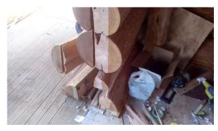
Figure 49: Splitting of bottom log weakened by vertical slot at door frame
