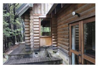
Figure 6: Two storey log house with slab on grade foundation
