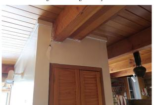
Figure 35: Typical cracking of gypsum plasterboard
