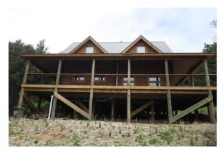
Figure 7: Two storey log house with pole foundation
