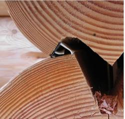
Here, in a window opening, you can see our gasket's 3 white fins, short, medium and long, and how they point down to, and seal against, the log below. The black rubber base is stiffer than the first fins. The gasket is stapled to the upper log only through the black base, and only in the gaps between the fins.
