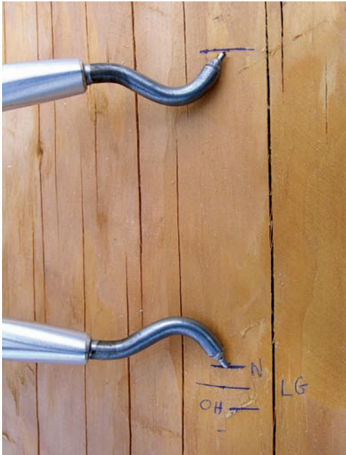
Figure 5.c: We use 3 scribe settings for each log. Always start by finding the long groove setting (LG), and scribing the groove. Then close down the scriber for the notch (N) setting (underscribe). Finally, open the scriber wider and scribe the flyways (Overhangs —OH).
