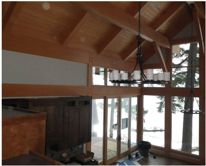
Fig.3.17 Cathedral ceiling and timber frame construction viewed from the inside of test house #3, Chase, BC.
