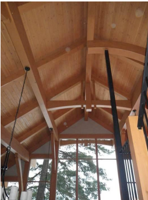
Fig.3.17 Cathedral ceiling and timber frame construction viewed from the inside of test house #3, Chase, BC.
