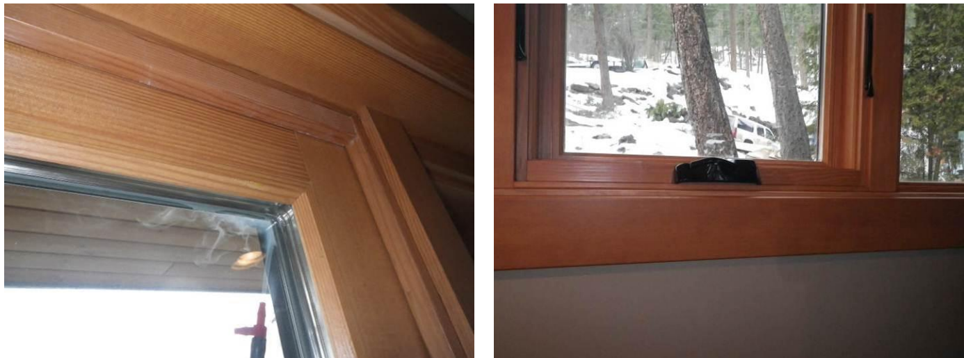
Fig.3.18 Smoke infiltration observed at sliding glass door between IGU and frame (left) and at operable window between sash and frame (right) under depressurization.
