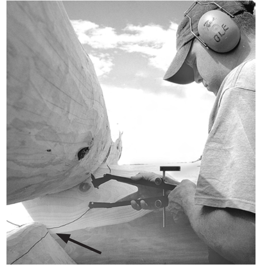
Figure 3: The groove is scribed, then the scribes are closed down slightly, and the notch is scribed. Perhaps you can see that the notch scribe line is a little above the groove scribe line—the difference in height is the underscribe amount for this notch.
