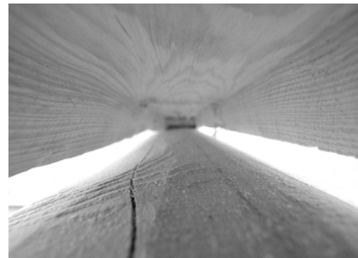
Figure 8: Looking down the inside of an underscribed long groove. No future hang-ups in sight here. There is a long, consistent-size gap in the groove of the log. The height of this little gap is equal to your underscribe amount.
