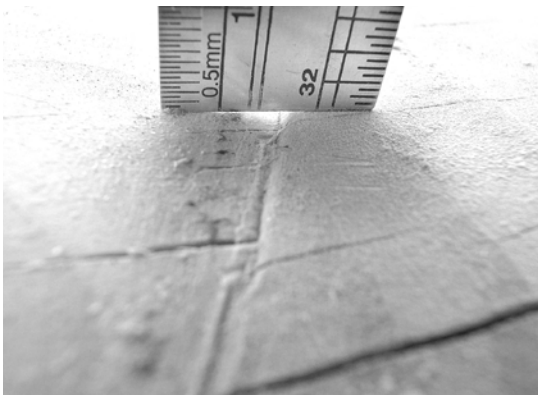
Figure 5A: A properly compressed saddle. The notch of the log above has compressed the wood of the saddle. This wood will rebound over time, and help keep the notch tightly fitted as the logs dry and shrink.
