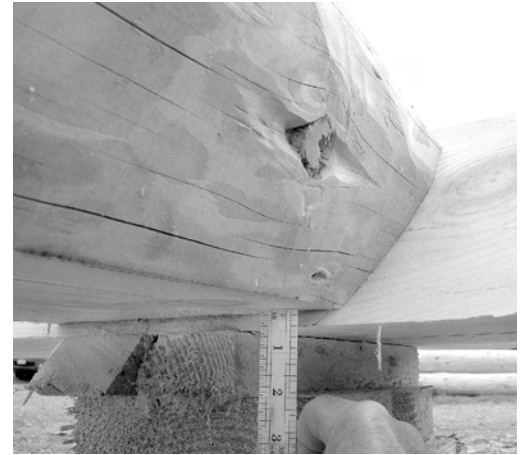
Figure 6A: Sill logs, showing the underscribe amount. For sill logs, the difference in height between the three-quarter-sill-log flat and the half-sill-log flat is the underscribe amount.
