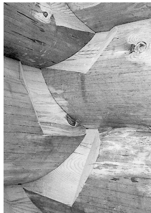
Figure 9: The shrink-to-fit, or Beckedorf “butterfly” notch. The saddle, instead of being flat or slightly concave, is convex—that is, the saddle is higher in the center. This is a photograph of a corner in the log home that I live in.
