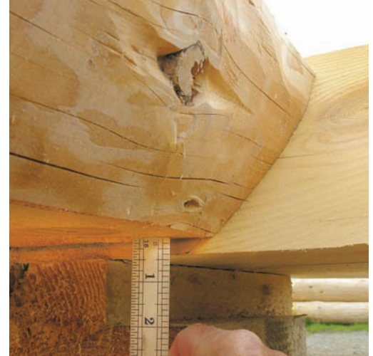
Figure 6.a: Sill logs, showing the underscribe amount. For sill logs, the difference in height between the three-quarter-sill-log flat and the half-sill-log flat is the underscribe amount.
