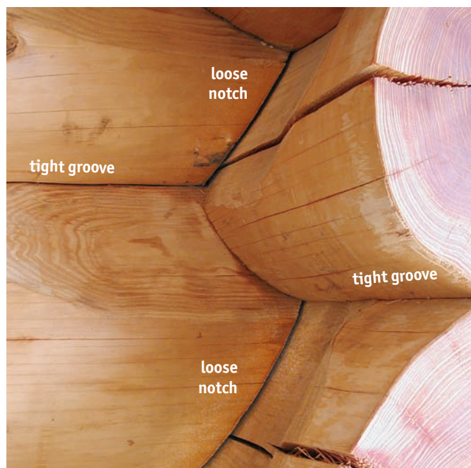
Figure 2: This building was not underscribed. As logs the logs dried, the long grooves stayed tight, while corner notches got gaps. The even width of the notch gaps prove that the scribing and cutting was carefully done: the gaps are not from poor craftsmanship, they're from normal and expected shrinkage. Underscribing solves this problem—underscribing helps keep the notches tight over time.
