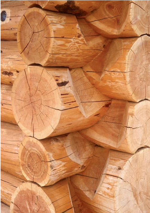
Figure 9: The shrink-to-fit, or Beckedorf “butterfly” notch. The saddle, instead of being flat or slightly concave, is convex—that is, the saddle is higher in the center.
