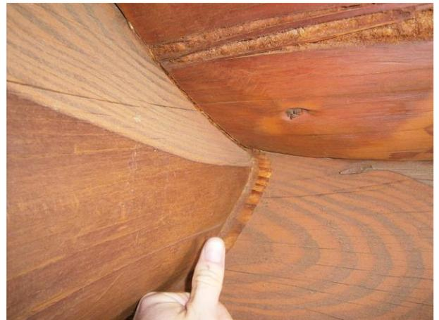
**Figure 22: Sliding of the logs at corners**
