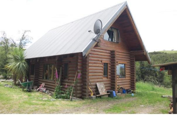
*Figure 3: Two storey log house with slab on grade foundation*
