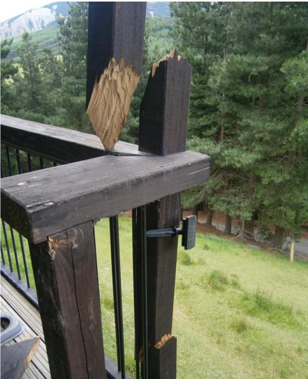
*Figure 25: Fracture of veranda post due to excessive lateral movement*
