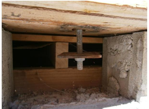
*Figure 27: Fractured tie rod*
