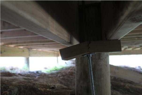
*Figure 32: Failure of timber anchorage block*
