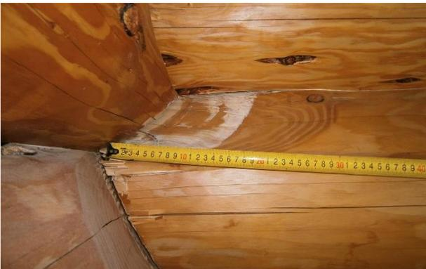
**Figure 42: Permanent deformation in corner area**
