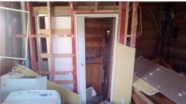
*Figure 54: Typical damage to light timber framing walls lined with plasterboard*
