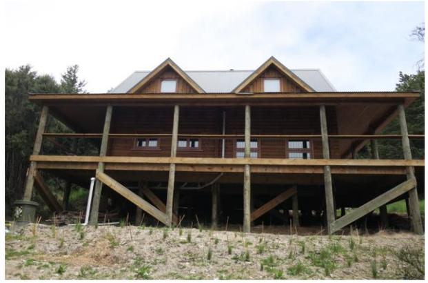
*Figure 7: Two storey log house with pole foundation*
