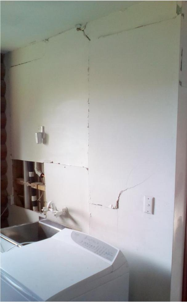
*Figure 36: Typical cracking of gypsum plasterboard*
