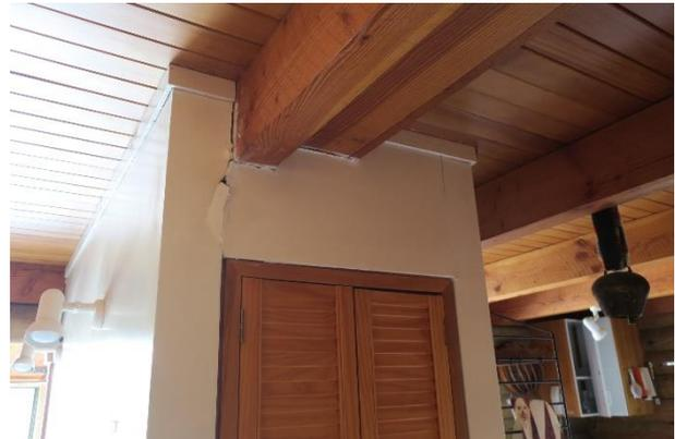
*Figure 35: Typical cracking of gypsum plasterboard*
