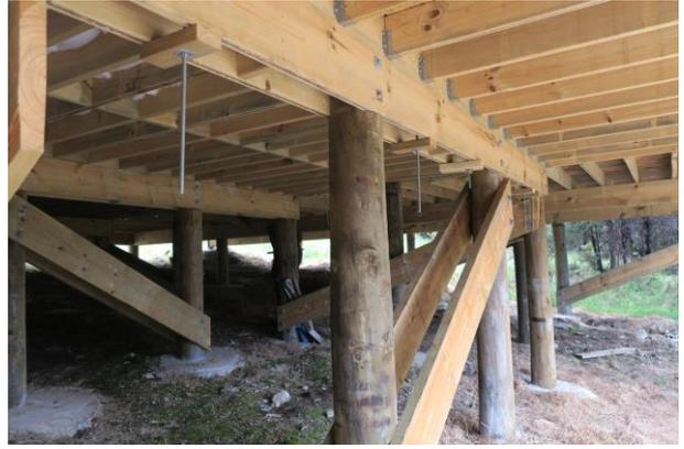
*Figure 8: Pole supports with diagonal sub-floor bracing*
