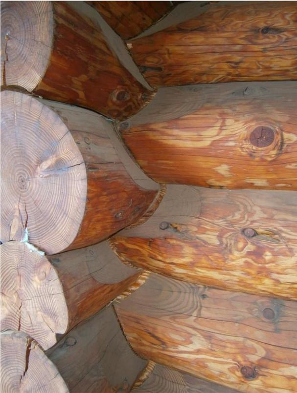
**Figure 41: Permanent deformation in corner area**
