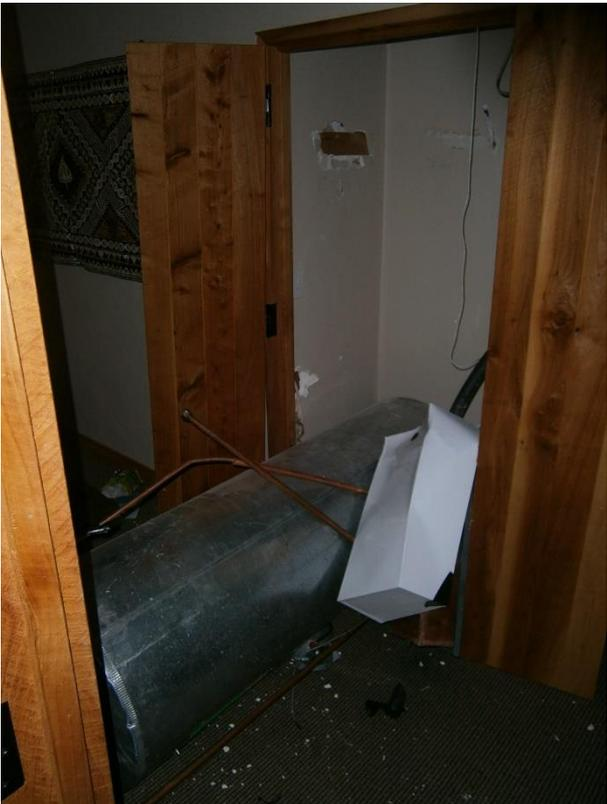
*Figure 37: Damage from insufficiently restrained water cylinder*
