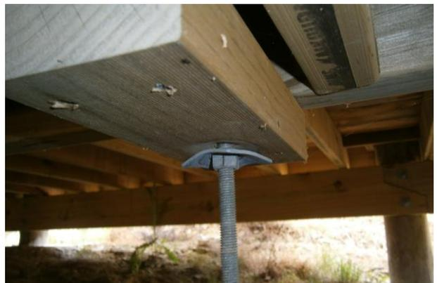
*Figure 29: Bent washer and wood crushing in anchorage block*
