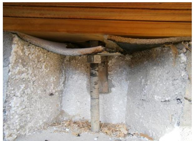
**Figure 45: Yielding failure or fracture of tension rod**
