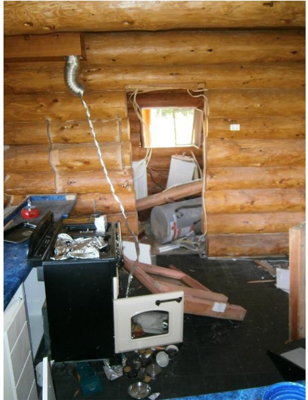
*Figure 55: Typical damage from falling or sliding of heavy objects*
