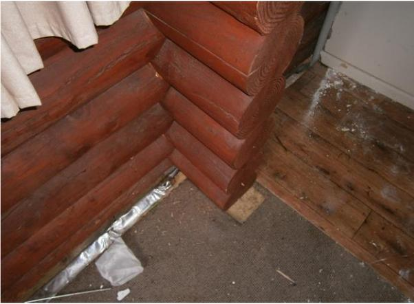
*Figure 24: Sliding of the logs on suspended floor*
