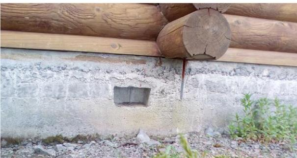
**Figure 12: Typical connection details with vertical steel rods and anchorage into foundation and half log (sill log)**
