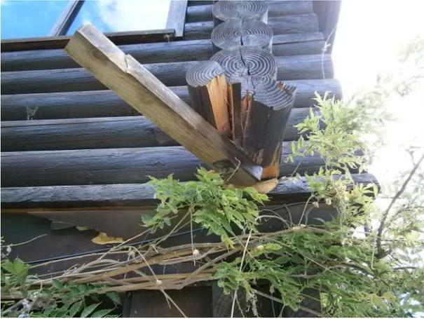
*Figure 31: Crushing of bottom log*
