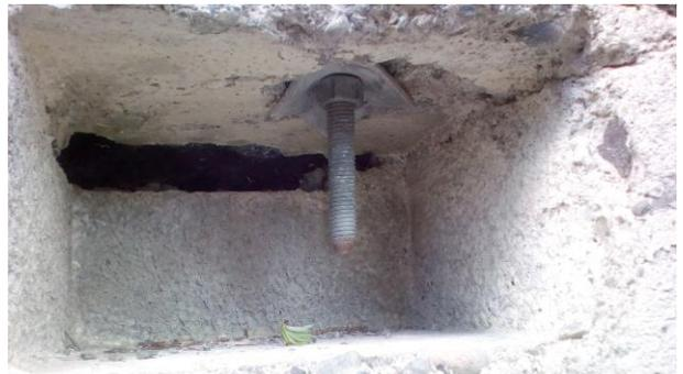
*Figure 28: Bent washer in concrete pocket*
