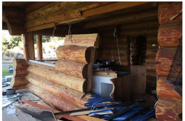
*Figure 50: Wall stability failure and splitting of logs*
